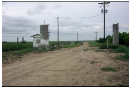
PHOTO 2 NORTH VIEW PUMP WELLS
