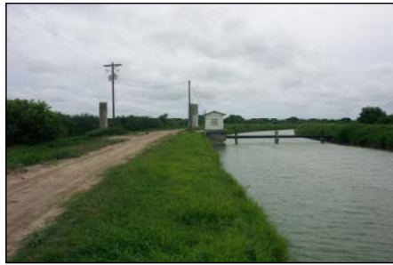
PHOTO 1 SOUTH VIEW ALONG CANAL
