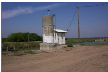
PHOTO 5 WEST VIEW PUMP WELL
